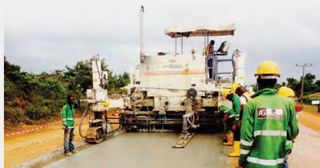
Construction of a concrete road at Apapa in Nigeria
