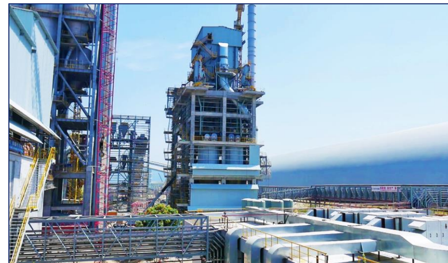
Pre-heater system cyclone at Okpella plant
