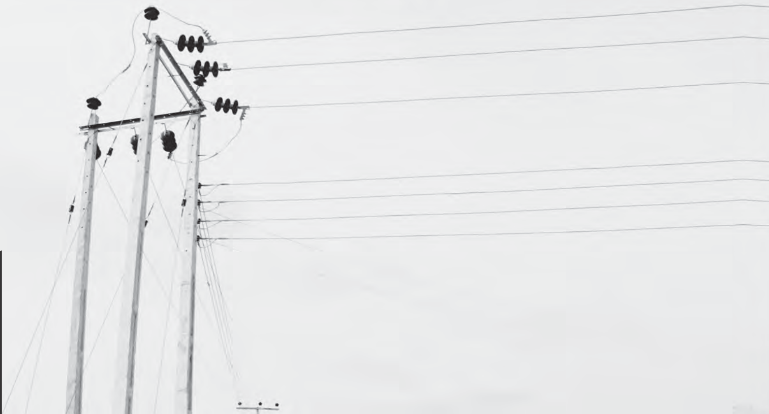
Construction and extension of low tension electricity lines to provide communities with access to low tension electricity from the installed transformers. The project entails erection of poles and extending low tension lines to Obajana, Apata, Iwaa and Oyo communities.
