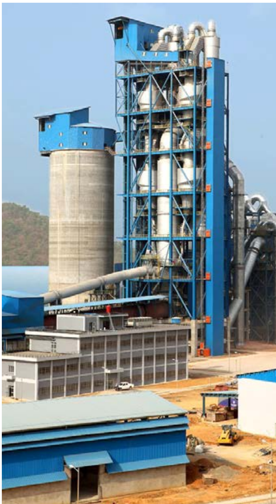
Dangote Cement's factories use modern pre-heater towers to improve fuel efficiency and reduce costs
